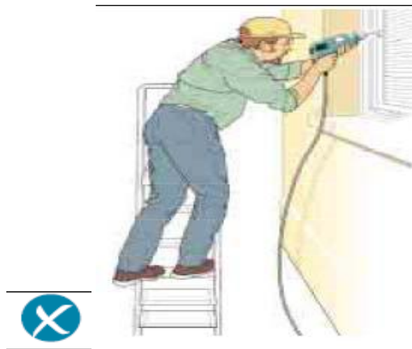
Incorrect – steps side on to work activity
